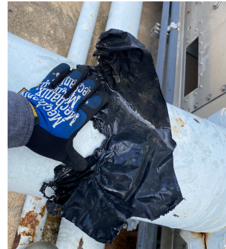
September 14: Suction Strainer clogged by debris
