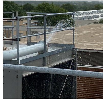
September 5: Gasket Failure
